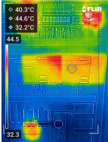
Monitoring Box are normal.
